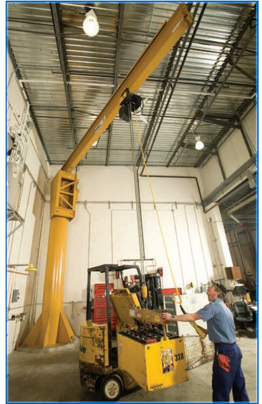
A Spanco Three-Ton Freestanding Jib Crane replacing motors
