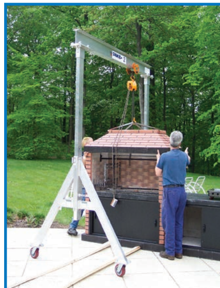
A 2-ton Spanco Aluminum Gantry Crane lifting the top portion of a grill for quick assembly.
