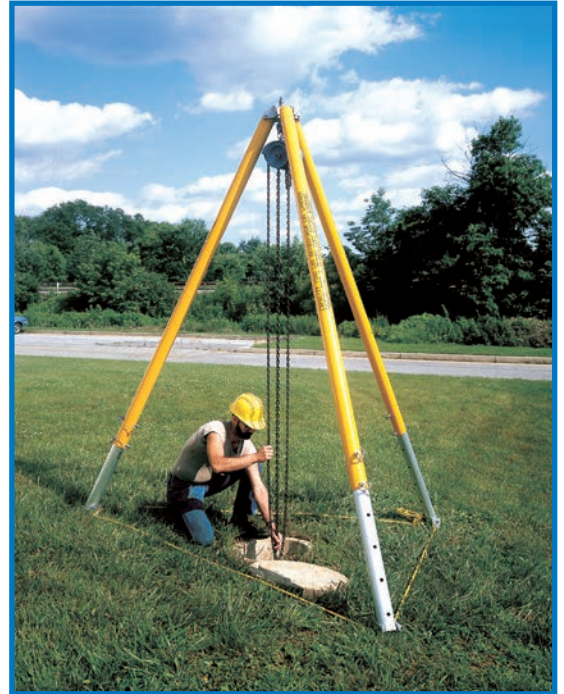
A worker using a Spanco Tripod with Mud Feet to lift a manhole cover single-handedly.
