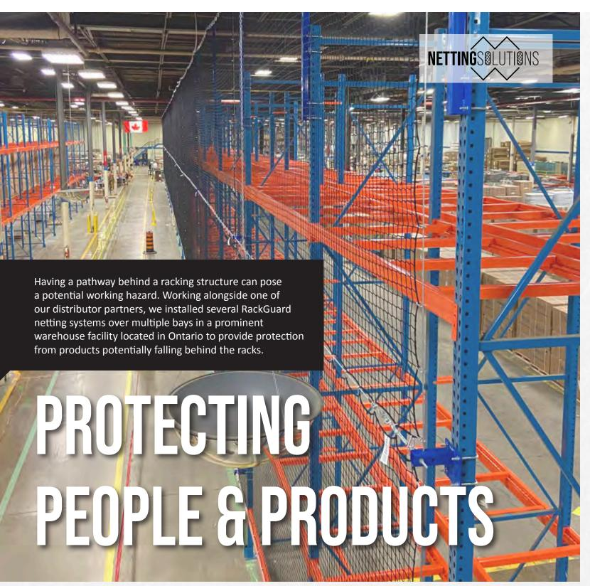
Our RackGuard system has been designed specifically for industrial racking applications. Each system utilizes engineered offset and extension brackets, custom sized netting panels, and cable systems to adapt to any racking configuration and maintain safety standards to create a soft catch solution that protects your racks, your products and your people. RackGuard systems meet OHSA, ANSI, NFPA and FDA standards for safety and engineered drawings are included with every installation.
